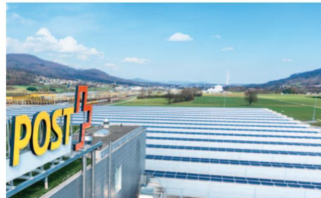
Swiss Post generates solar electricity for its own use in its photovoltaic systems. The surplus is fed into the public grid.
